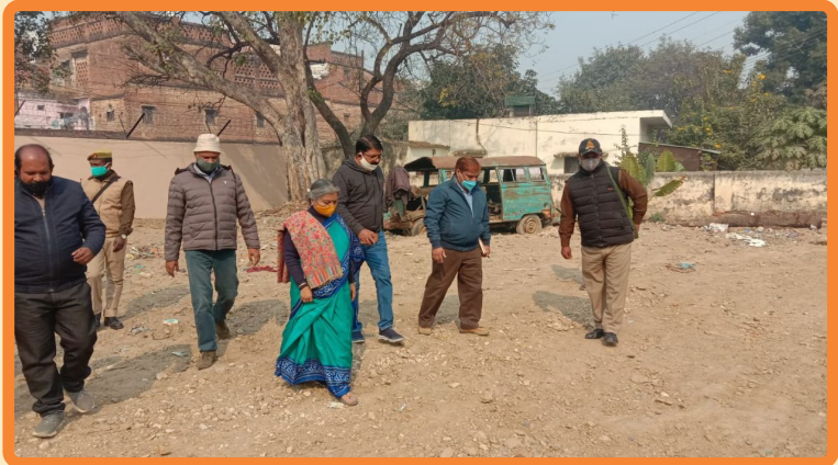
Hon'ble Vice Chancellor inspected the Badminton Court under construction in the Student Activity Center complex.
